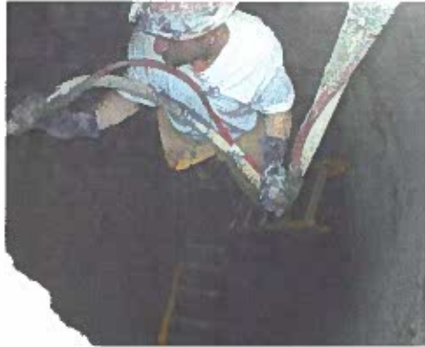
Spraying of Cementitious Mixture
