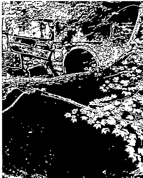
Photo 2: Musquash Road – Culvert Outlet
