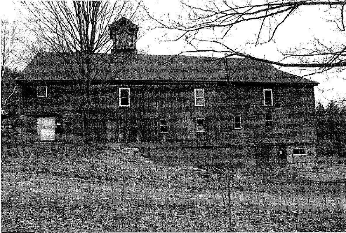
Figure 5. North elevation. Photograph by John Butler. (November 7, 2002)
