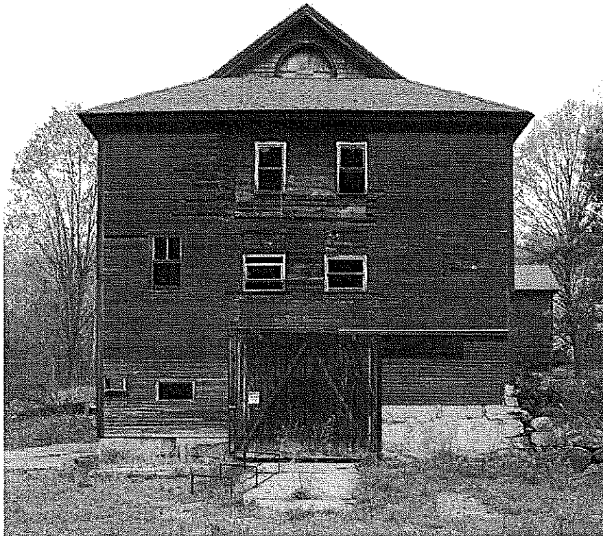
Figure 7. West elevation, silo ell to the right. Photograph by John Butler. (May 15, 2003)
