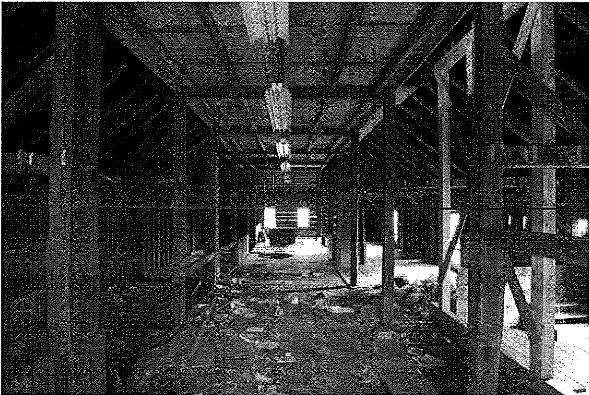
Figure 8. Drive bay looking west. Photograph by John Butler. (May 15, 2003)
